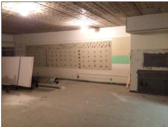
Tackboards, Ceiling, & Flooring Removed
