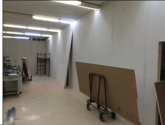
Temporary Wall Separating Kitchen Construction Area from Cafeteria
