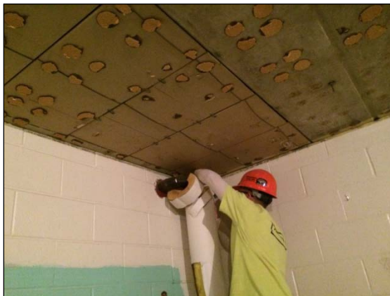
Removing Pipe Insulation
