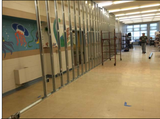
Temporary Wall Separating Kitchen Construction Area from Cafeteria
